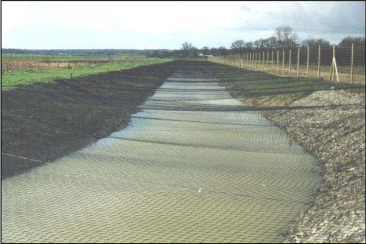
Cleared and netted drainage channels offer no bird attraction whilst maximising their drainage functions
