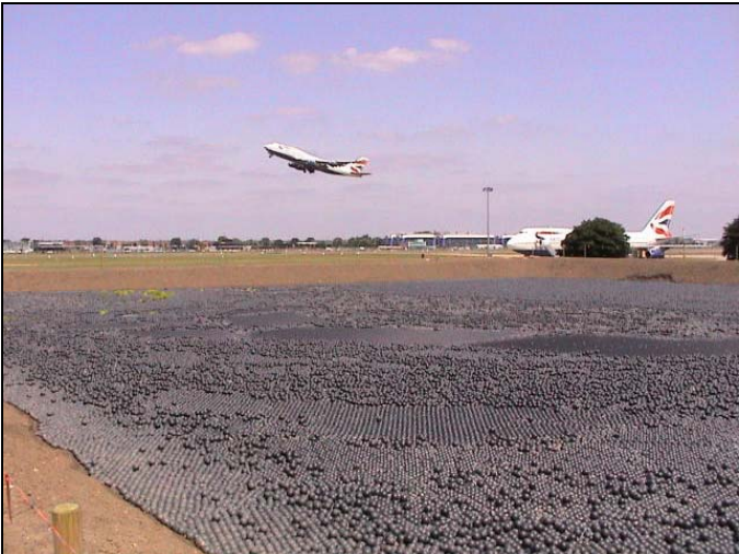
Water retention ponds can be proofed against Birds with netting or, as in this case with floating 'bird balls'
